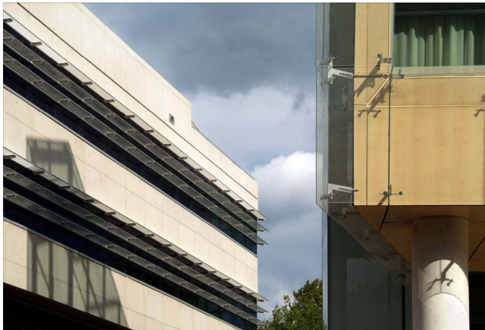
Figure 4A. Comparison of the North and South Building exterior cladding
