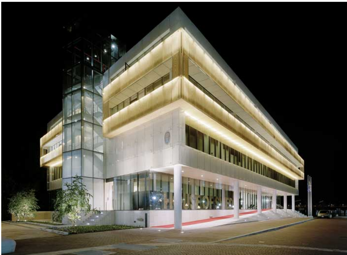
Figure 2A. Night view of the North Building
