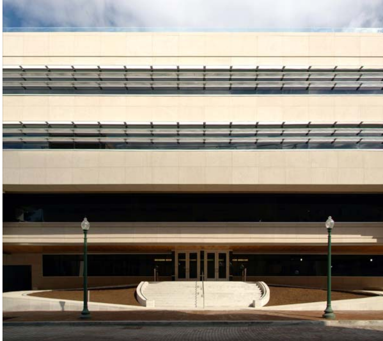
Figure 3A. Picture of the South Building
